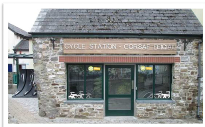
Photo Above; Haverfordwest Cycle Station
